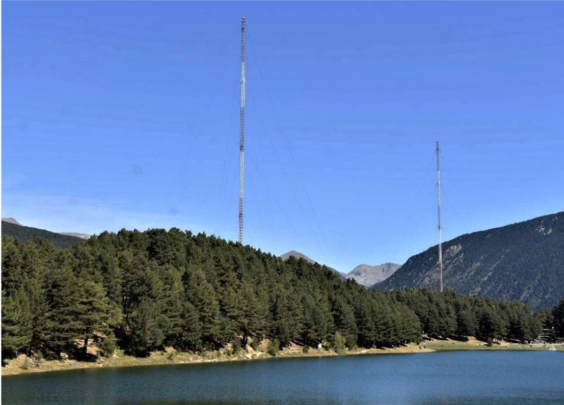
*left: the 2 masts were linked to the Encamp transmitter by two 1km feeder lines. Last frequency being used before its closure in 1981 was 702 kHz.*
