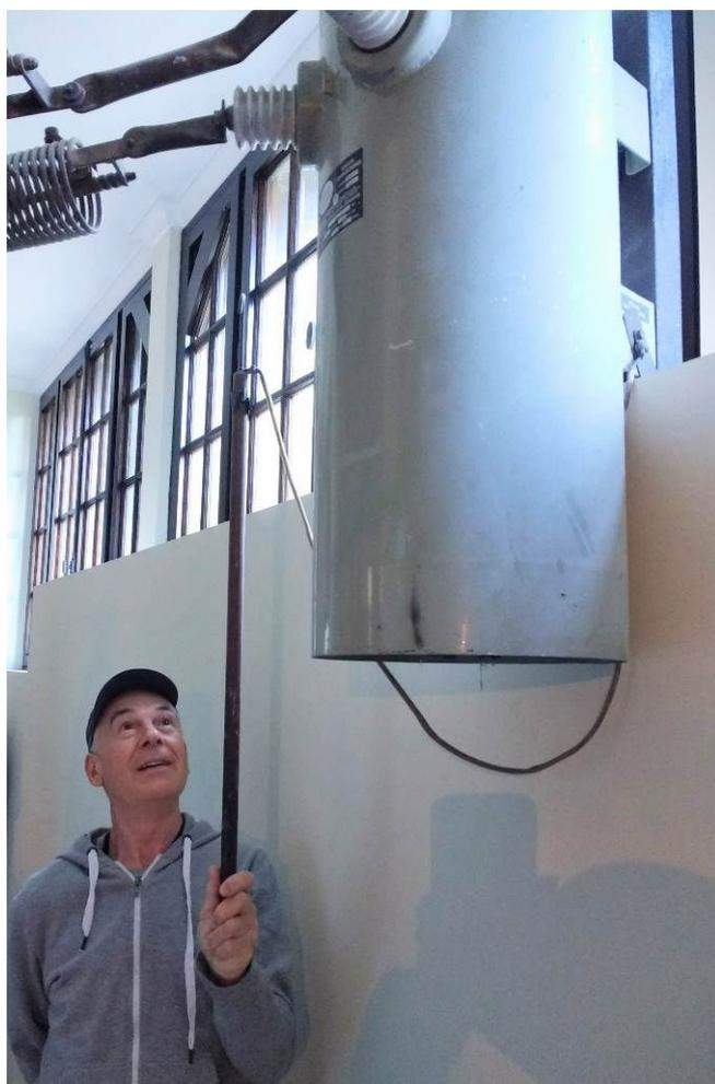
*left: turret on Radio Andorra transmitter building. right: Dave Kenny with balun transformer at Encamp.*
