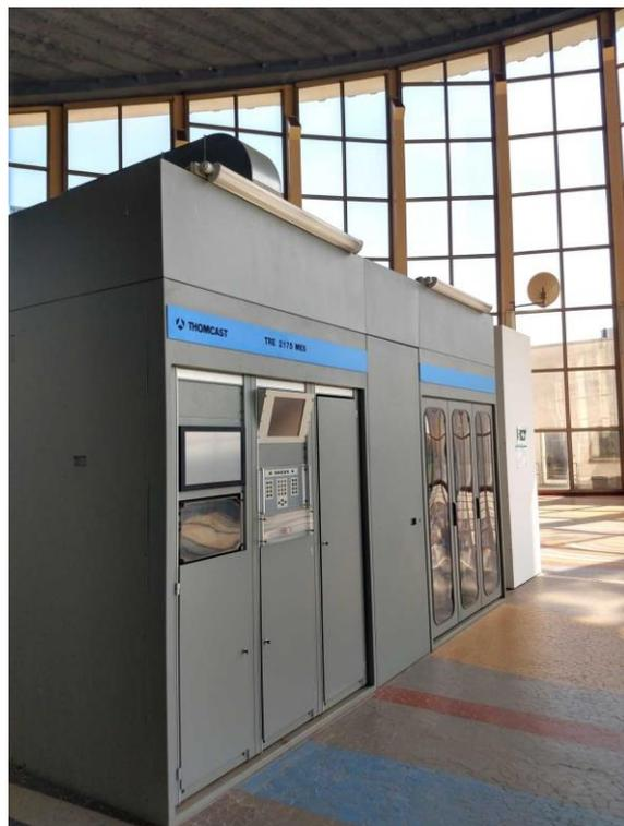
We toured the old transmitters still in situ in the building. Originally operating with 400 kW on 182 kHz, adjusted to 180 kHz in 1960, with power increased to 2 megawatts in 1976, with frequency 183 kHz from 1978. BCE had replaced the 1975 valve transmitters in 2015 with transistorised transmitters housed in a
