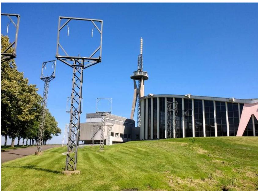
The re-enforced concrete tower next to the transmitter hall was originally used for the Telesaar TV channel. Now, since November 2020, it has been used by Saarländischer Rundfunk to radiate digital TV and DAB+ radio signals.
