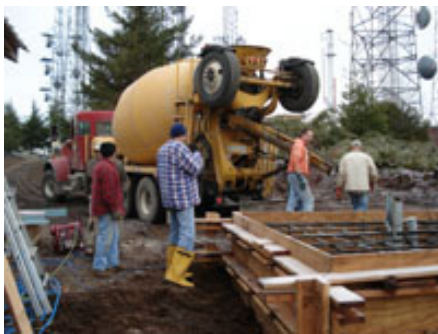
Bauarbeiten (Photo Glenn Gately)
